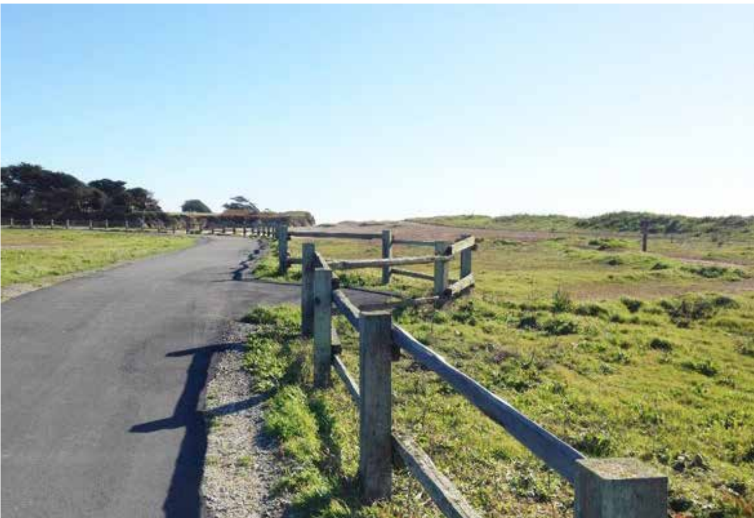
SPLIT RAIL FENCING (COUNTY STANDARD)
